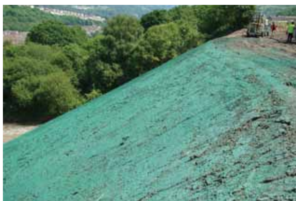
The application of our HydraMax hydraulic mulches will work with a wide range of mechanically agitated hydroseeding equipment, and the decreased water to mulch mixing ratio will get your job done faster.
