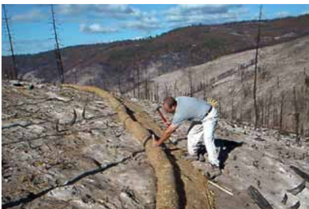
Steep Slope Protection and Sediment Control, Washington, USA
