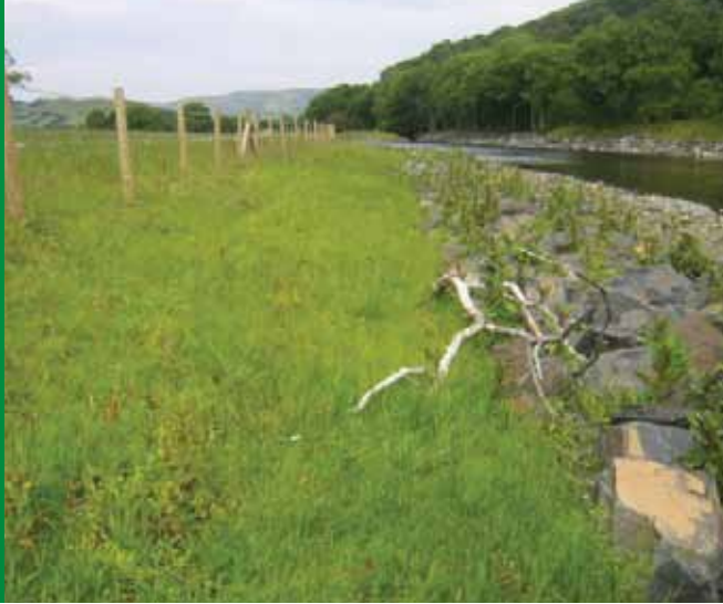
Vegetation establishment through VMax® P550® six months after installation, UK.
