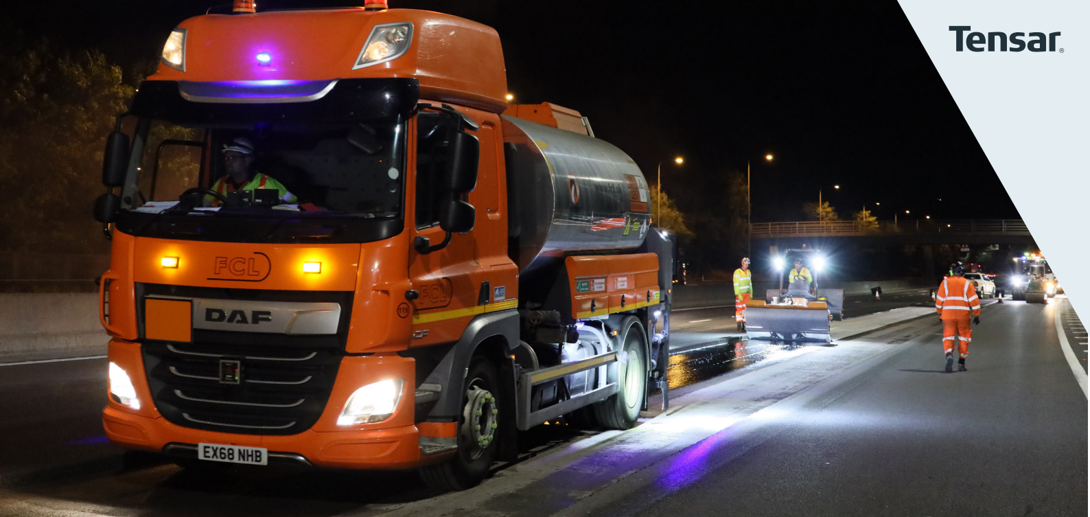
Installation of Tensar Glasstex P100
