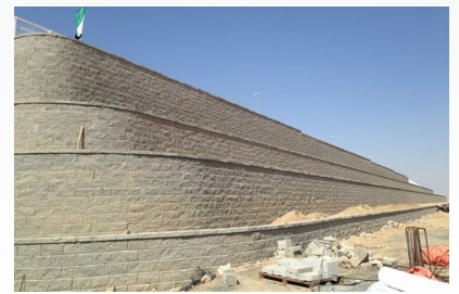
Tiered Tensar reinforced soil walls with modular block facing
