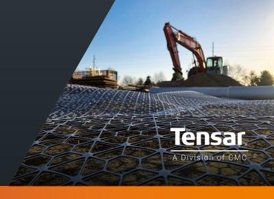
This Installation Guideline provides a step by step guide for Contractors installing Tensar® InterAx® geogrid supplied by Tensar® International or any of its appointed distributors. The guideline applies to both the permanent and temporary mechanical stabilisation of areas over which vehicular access is to be provided.
